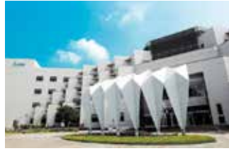
Tainan Plant (Diamond-rated Green Building)
