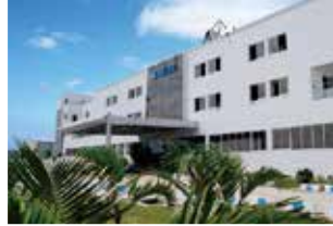
Rudrapur Plant (Green Building)
